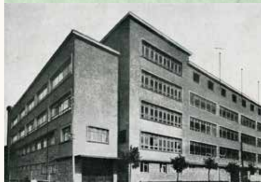
The German High School, 1934. Today the building houses the National Academy of Music.
