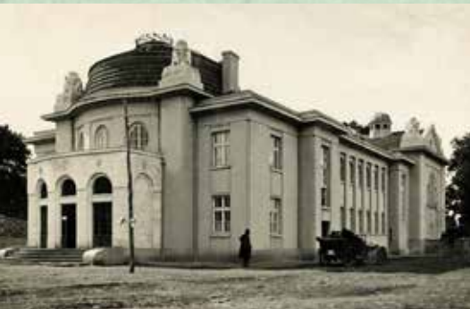
Gorna Banya – the new modern mineral bath, built between 1922 and 1927
