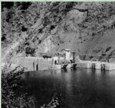
The dam on the Iskar river and the power plant near Pancharevo
